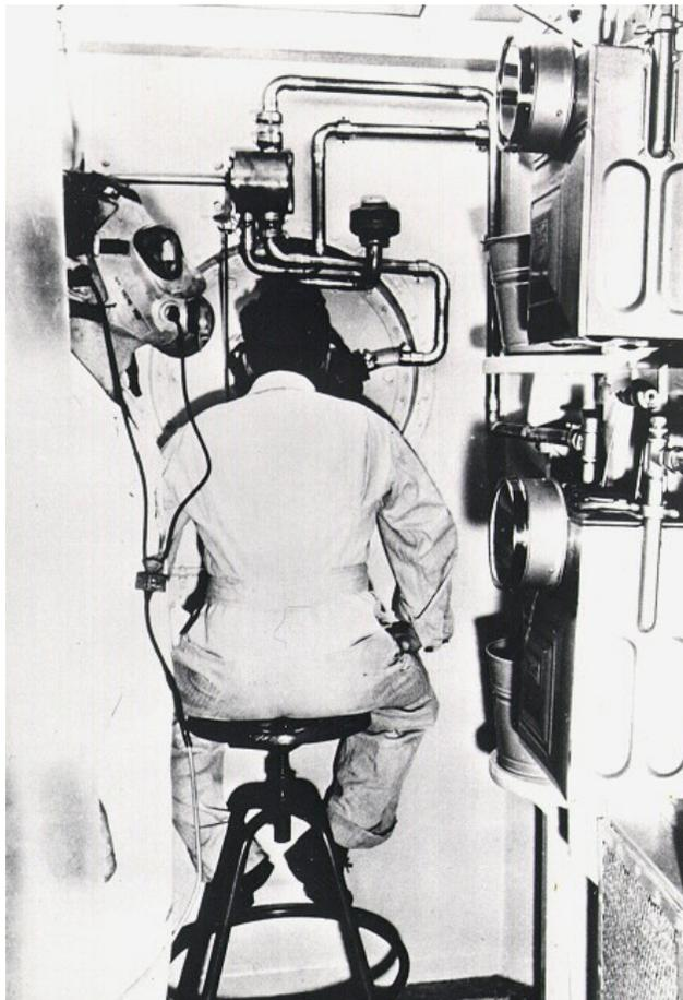
**The one-million-liter test sphere, nicknamed the “Eight Ball,” was a cloud chamber used to study static microbial aerosols. During Operation Whitecoat, the volunteers breathed metered aerosols of Q fever or tularemia organisms through ports along the perimeter of the sphere.**
